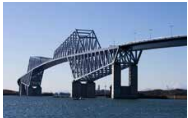
Tokyo Gate Bridge – 2012 - Japan
